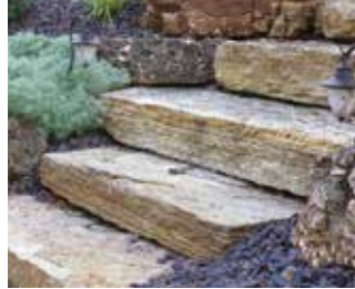
Weathered Limestone Irregular Step
