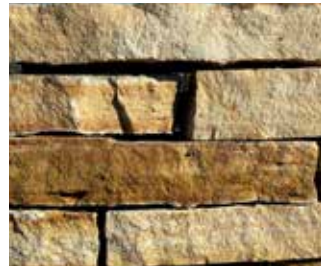
Alpine 8" Drywall 2 - 3" & 3 - 4" Thick
