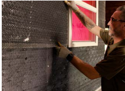
REPEAT TO TOP STAGGERING SEAMS
